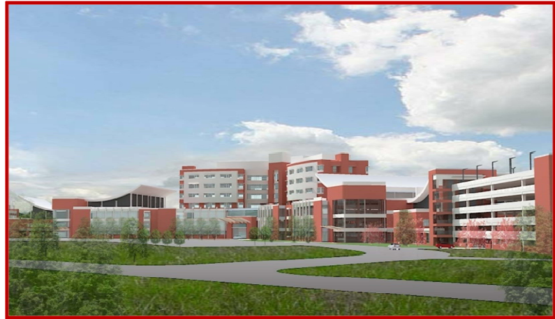
The New Community Hospital, Fort Belvoir, VA Credit: HDR Architecture, Inc.
